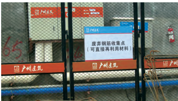
Collection point of scrap reinforcement bars (directly reusable materials)
